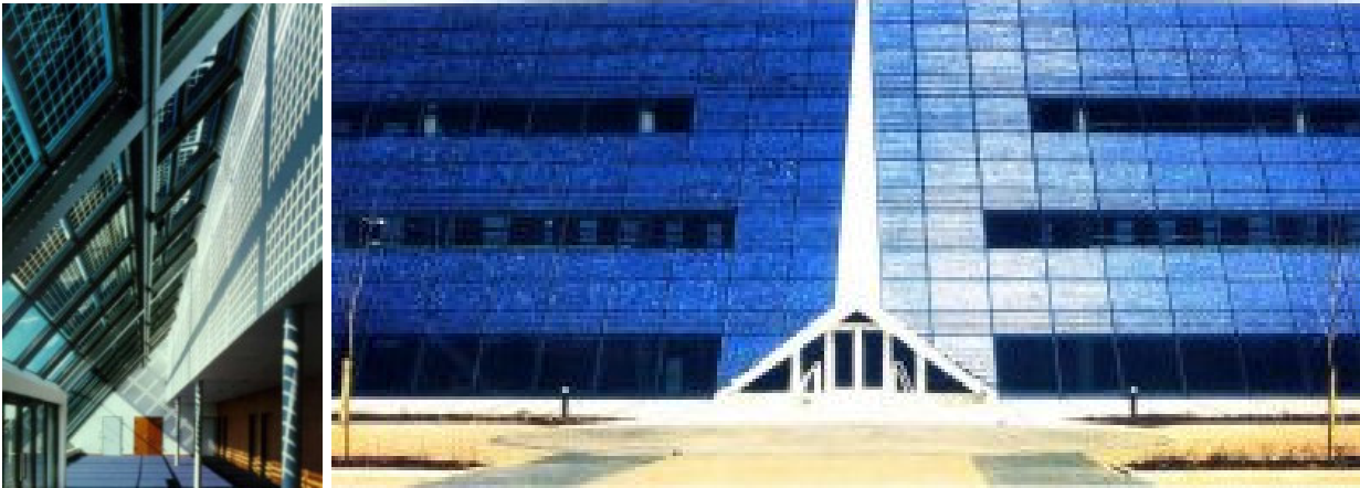
Atlantis and Prosol Solar PV Facade
